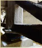
TOP Isolators at the base of each primary structural column allow the building to move independently from the shaking ground during an earthquake.
