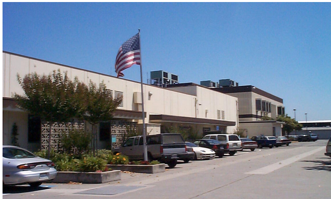
Existing Laboratory Remodel
